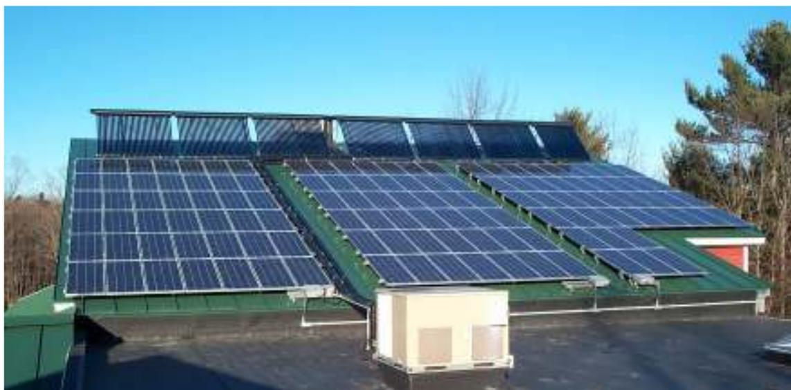
**MHF's 202-tube solar hot water system (angled tubes at top) & 15 kilowatt solar electric array.**
